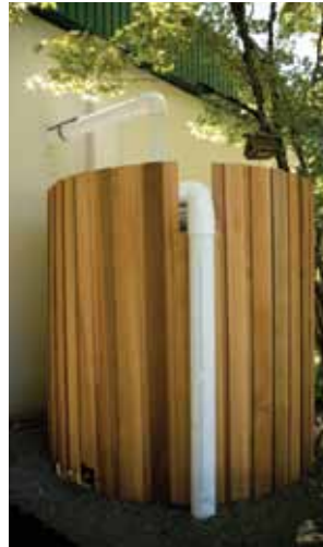
Rainwater capture tank provides water for lawn
